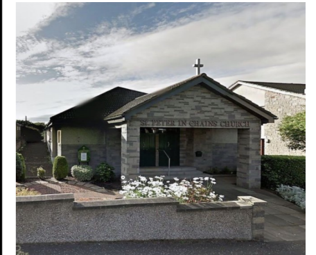
St Peter in Chains Church, Inverkeithing
