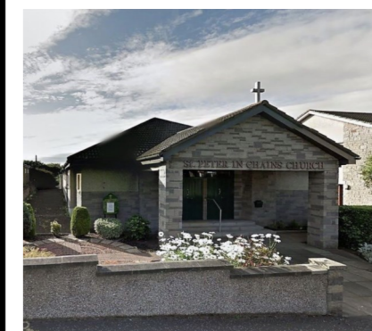
St Peter in Chains Church, Inverkeithing
