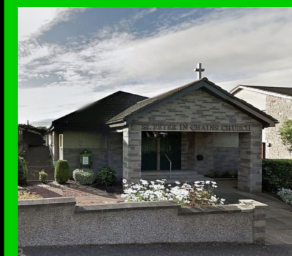
St Peter in Chains Church, Inverkeithing
